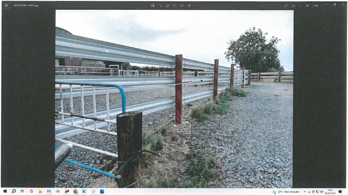
Boundary to run from wood post and continue 1 m. North of steel fence
